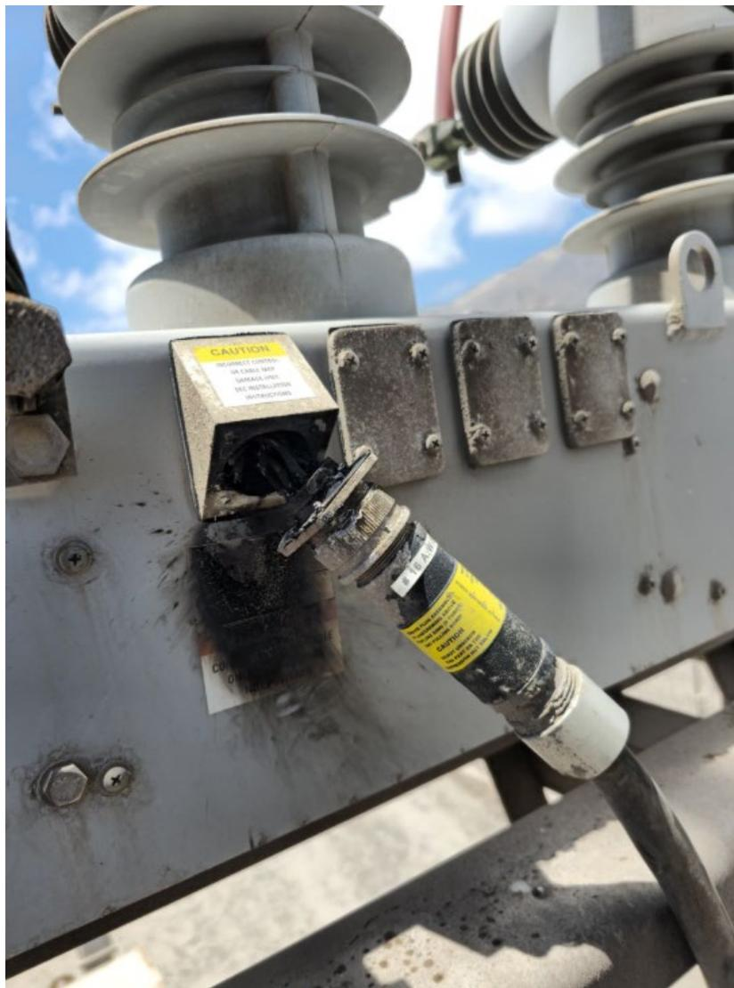
DAÑO EN EQUIPO PRIMARIO 52ET3, PRODUCTO DESCARGAS POR AVE EN ESTRUCTURA SUPERIOR 52ET3
