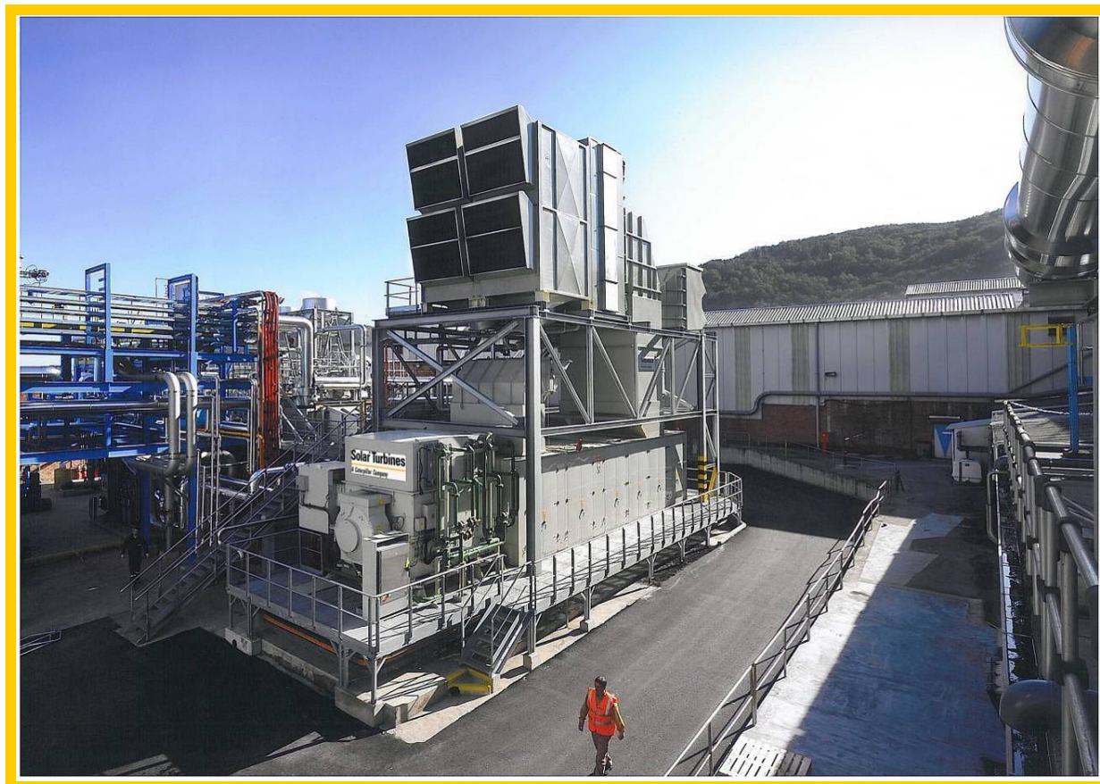
One (1) Titan 250 Gas Turbine Generator Set For CMPC - Talagante
